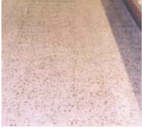
Fig. 6: Polished concrete surfaces serve a decorative function, while allowing moisture vapor to escape
