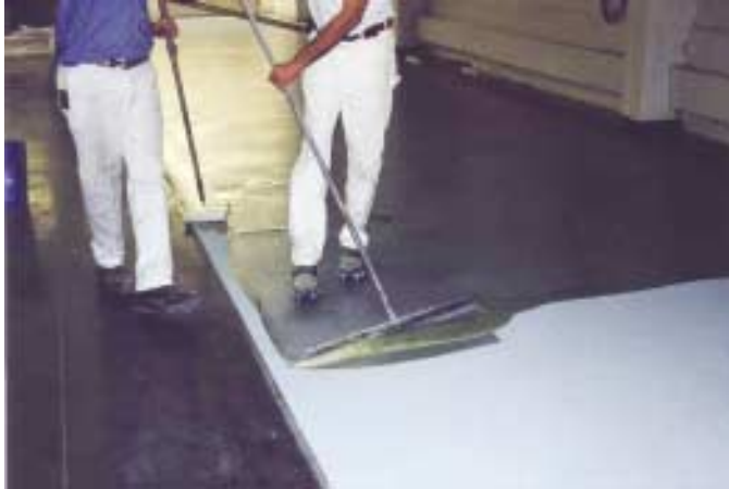
Fig. 4: Special epoxy- and copolymer-modified cementitious overlays are used as a separation layer between the base concrete and the applied flooring system (photo courtesy of Liquid Plastics)
