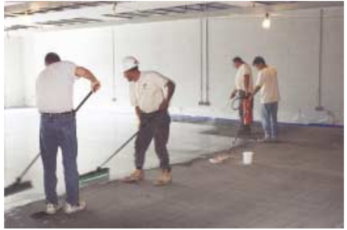
Fig. 3: Moisture-retarding acrylic or specialized epoxy coatings slow moisture emission from the slab and help isolate the applied flooring material from the pH-raising effects of soluble alkalis in the concrete (photo courtesy of Koester America)
