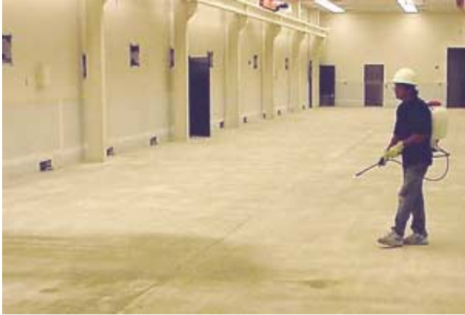
Fig. 2: Spray-applied reactive penetrants combine with alkalis within the concrete, reducing the pH and permeability to moisture vapor (photo courtesy of SINAK Corp.)
