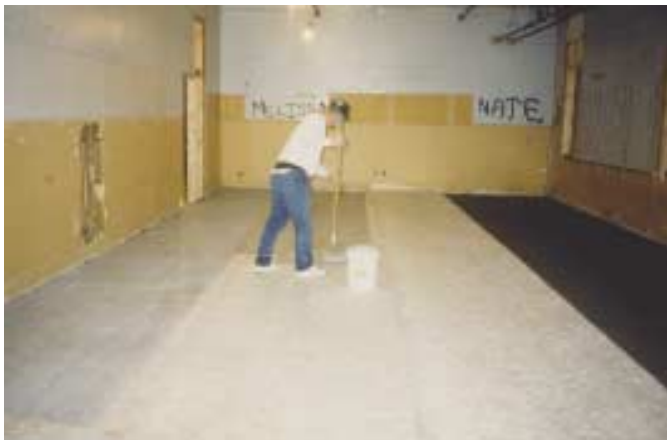
Fig. 5: Fiber mat membrane can be adhered directly to a prepared concrete surface or applied over certain penetrants and approved coatings to provide a moisture diffusion path
