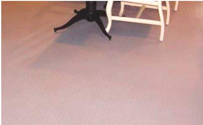
Fig. 8: Some nonadhered, interlocking tiles can be used when high moisture emission levels are present. Concrete beneath the tiles must be shotblasted to open the surface so any moisture condensing beneath the tiles can be reabsorbed by the concrete (photo courtesy of Flooring Adventures)
