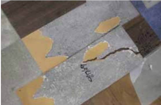
Fig. 5: Bond performance of various flooring materials and adhesives were used to verify that the new concrete mixture would perform as required
